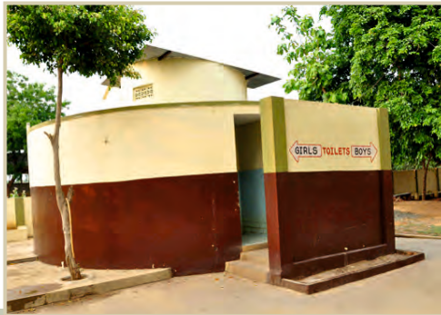
WASH ROOM FACILITY
